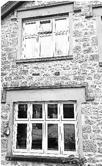
Figure 6: Contemporary image of the north elevation of Ivyleigh showing the decorative window headers
